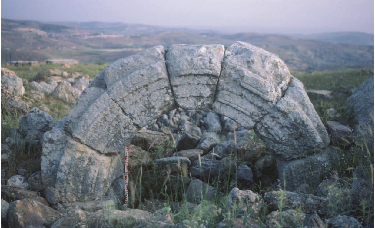
Fig. 13. Wall (row of arches) H: north face of arch f. Photo F. Villeneuve, 1983, looking south.
