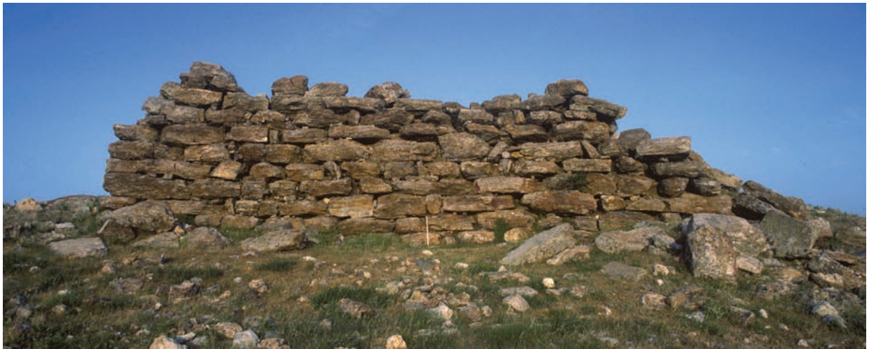
Fig. 10. Qasr, west wall (B), from outside. Photo F. Villeneuve, 1983, looking east.
